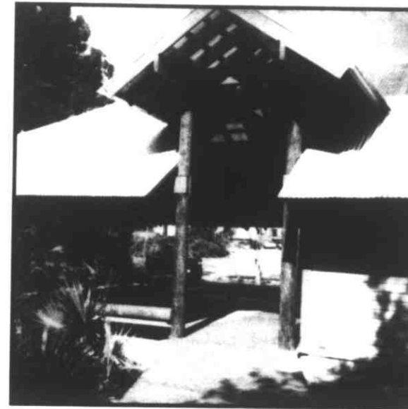
The Nature Center building at Hoo-Hoo Park is complete. It is 3000 square feet and has all electrical and water services.
